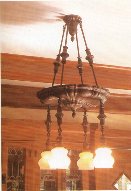
233. Brass dining-room ceiling fixture suspended on chains and with four frosted-glass shades, c.1910, Echo Park (Los Angeles), California. This popular dining-room fixture style is closely related to the "shower" variety, which placed its bowl-shaped element flush to the ceiling as a backplate for multiple chain-hung lights. Painted wood graining is seen behind it.
