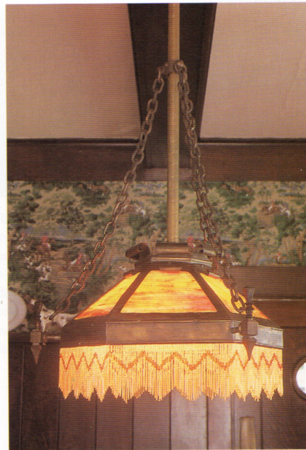
236. Brass and art-glass dining-room ceiling fixture, suspended from a rod and chains, 1910, Spokane, Washington. Converted from a combination gas and electric fixture, finials now indicate where the gas jets were. Glass-beaded fringe shades the glare of concealed electric bulbs.
